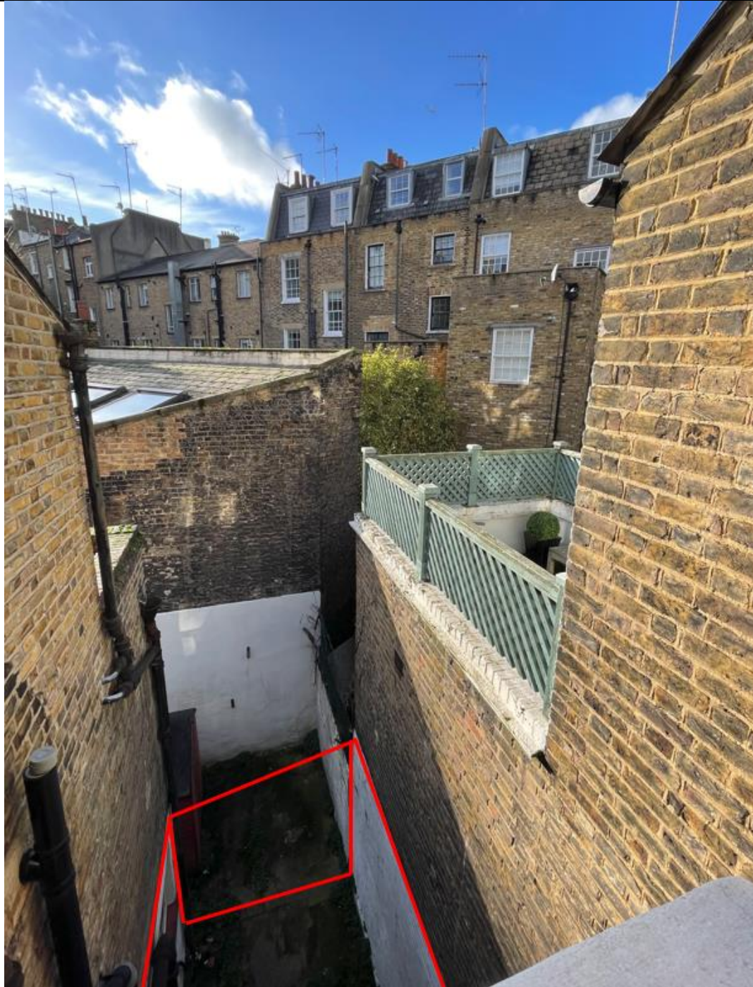
Rear of 11 Churton Place with approximate position of proposed extension indicated in red
